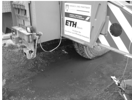
Figure 2. 2D-laser scanner mounted underneath the crane.
