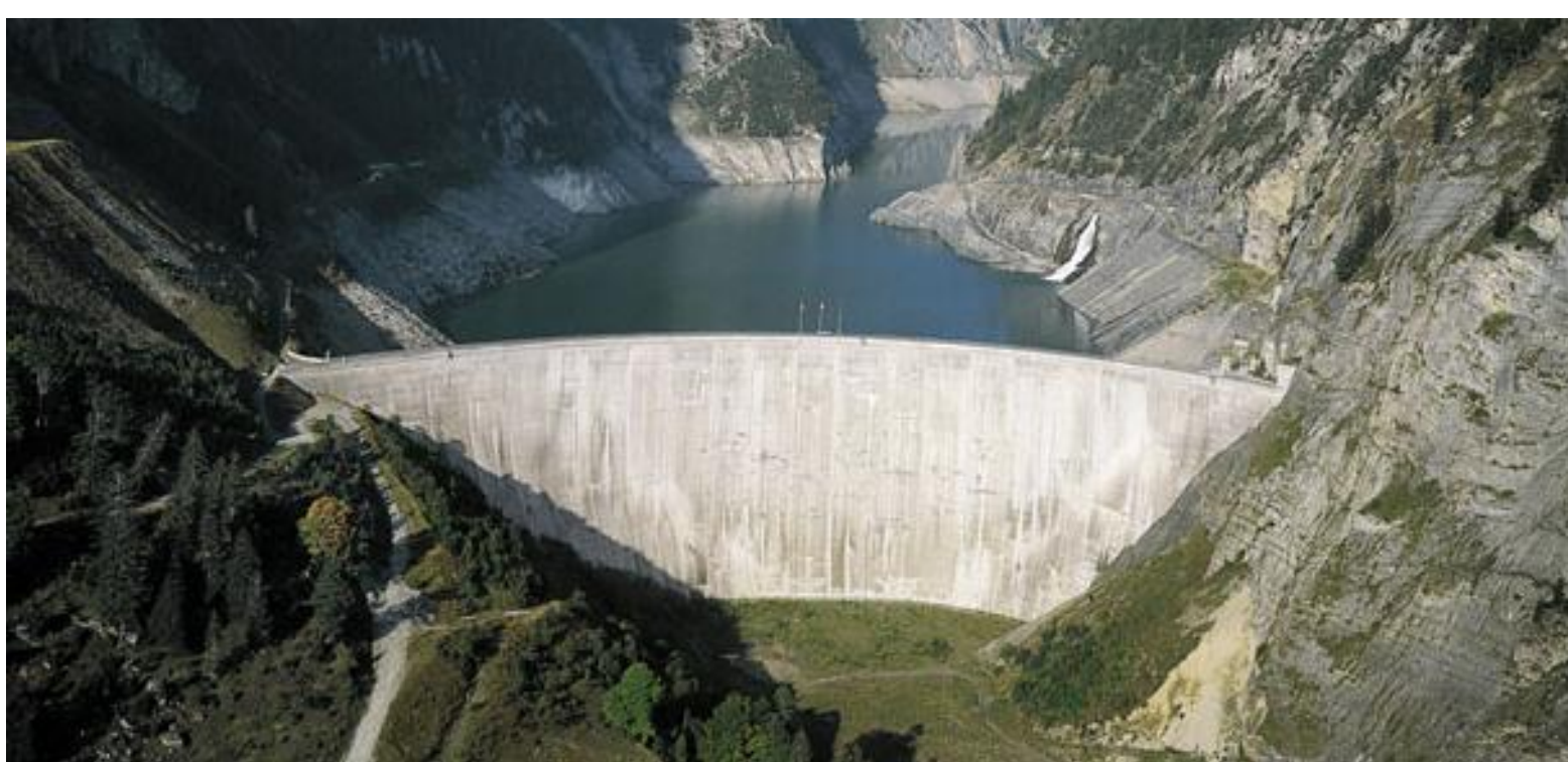
Abb. 1: Staumauer Gigerwald [axpo]
