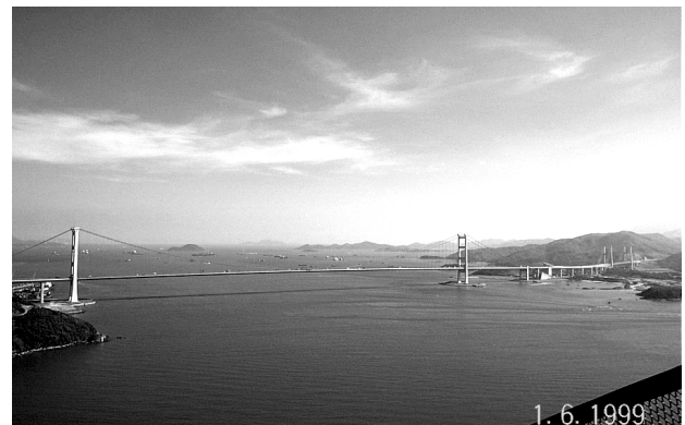
Fig. 10. Tsing Ma Bridge (Hong Kong)
