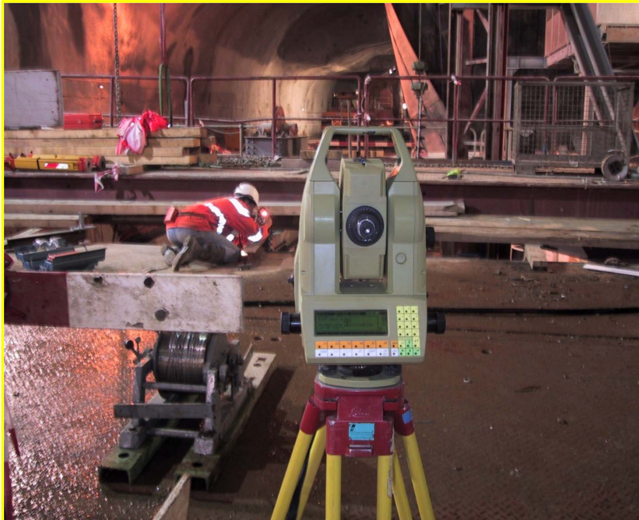
Measuring plumb lines on top
