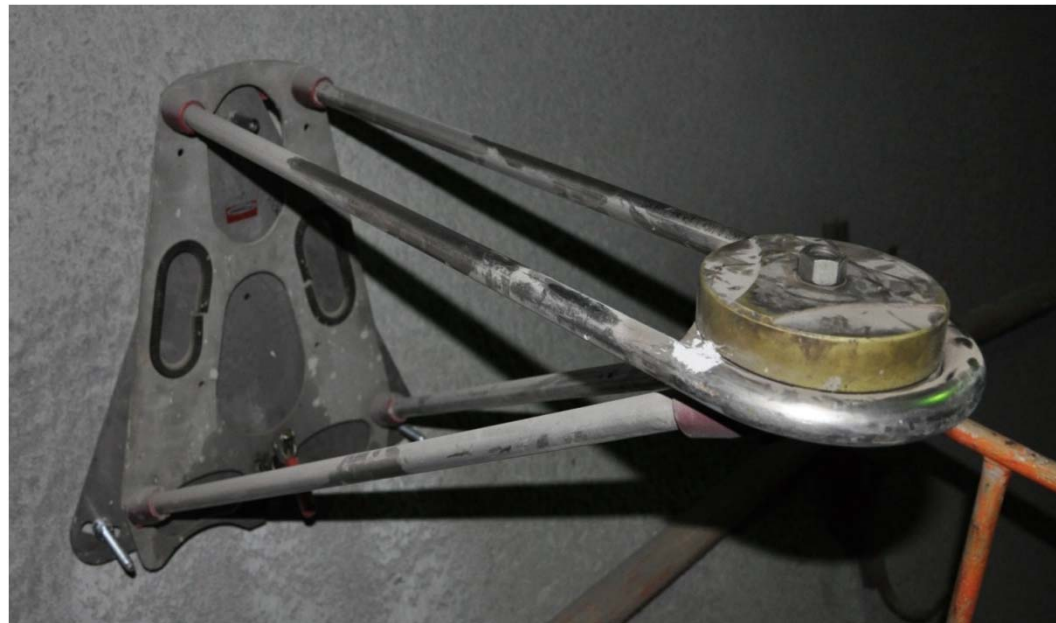
Losatec mounting system in Gotthard Basetunnel near Faido. Source: Stephan Schütz
