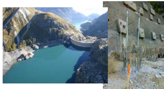
Dams and Retaining walls
